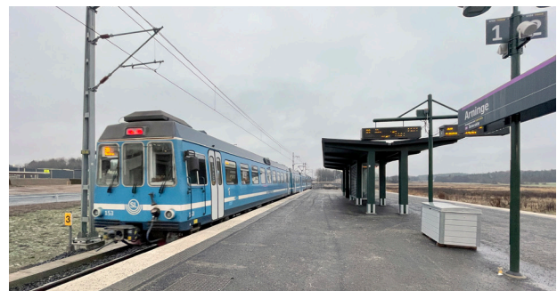
▲ Thyristor controlled rectifier manufactured by PLUTON at Arninge substation (Stockholm, Sweden)
